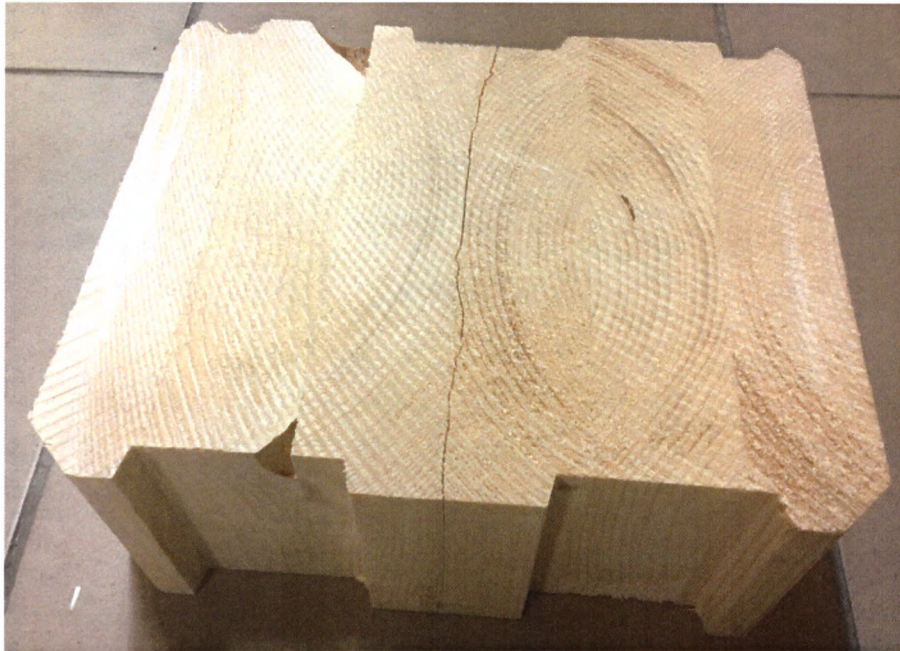
Picture 4. Damage of the sample LL/404/19/04
